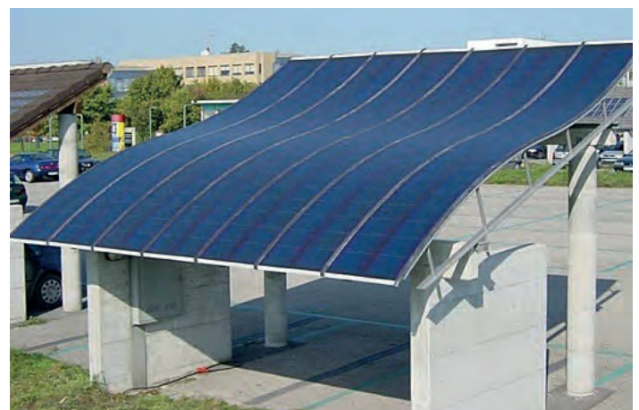
Figure 5 Example of in-roof mounting of flexible PV modules. Image courtesy of Solar Constructions ( www.solar-constructions.com )
