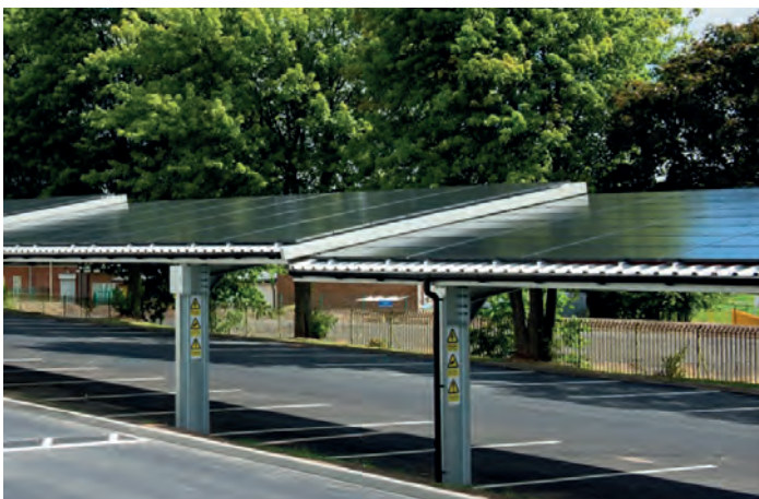
Figure 2 Example of on-roof mounting of framed PV modules. Image courtesy of Evoenergy ( www.evoenergy.co.uk )
