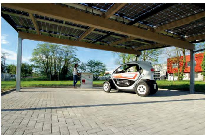
Figure 4 Example of in-roof mounting of glass-laminated PV modules. Image courtesy of Si-Module ( www.si-module.com )
