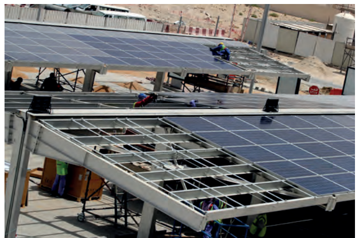
Image courtesy of Enerwhere Sustainable Energy DMCC ( www.enerwhere.com )
