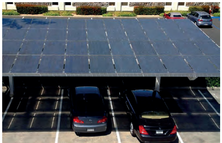
Figure 3 Example of in-roof mounting of unframed PV modules. Image courtesy of Sunpreme ( www.sunpreme.com )
