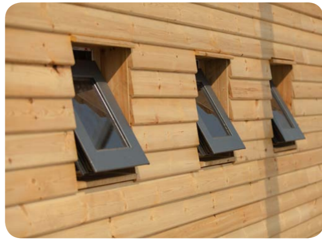
Locally sourced timber weather boarding
